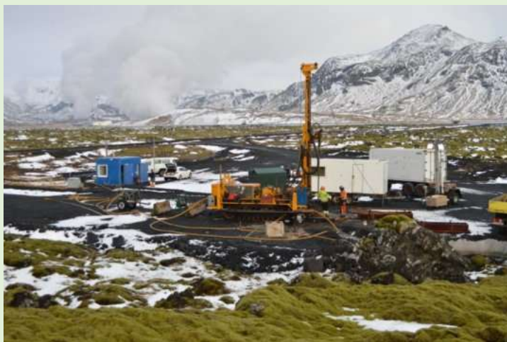
CarbFix I pilot CO 2 injection site during wireline diamond drilling to recover a 150 m of core from the CO 2 storage reservoir in 2014 (~2 years after CO 2 injection). Steam emissions from the Hellisheidi geothermal powerplant are visible in the background. Credit: Photo by Juerg Matter
